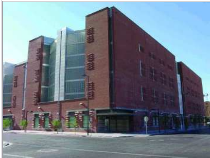
The 4th Avenue Jail runs the edge of the sidewalk on all sides. The V-shaped wall of glass block brings ventilation and light to the otherwise windowless interior.
