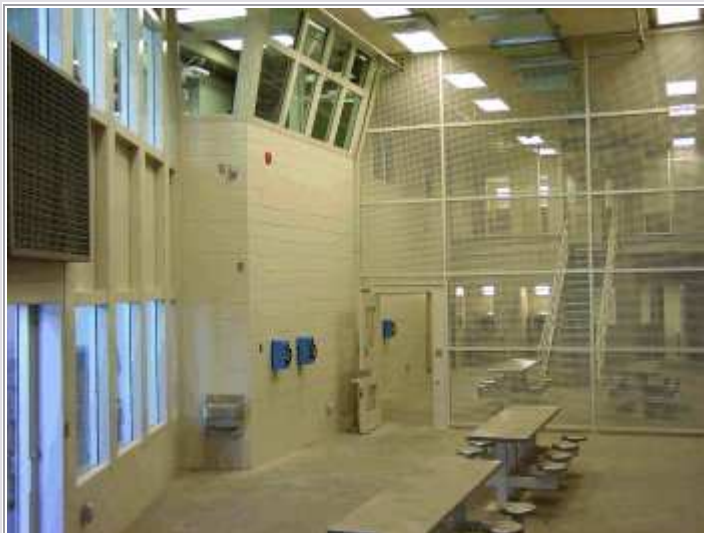
Security mesh fully segregates this 72-bed unit by two halves, monitored by a single control room on the mezzanine. PHOTO CREDIT: Sgt. Artur Fay
